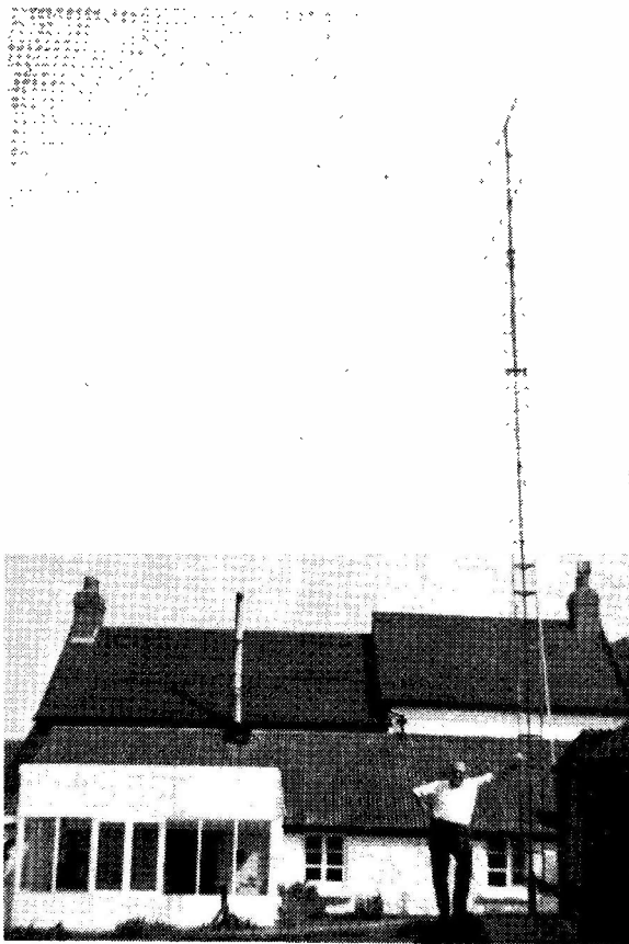
Neat two-metre beam assembly on its home-constructed lattice tower at G3KDG, Petrockstowe, South Devon. The beam is a slot-fed six-over-six and, remote as he is, most of G3KDG's contacts at any sort of distance are on CW. He has worked G3DAH (Herne Bay, Kent) on numerous occasions, always with a good signal.
